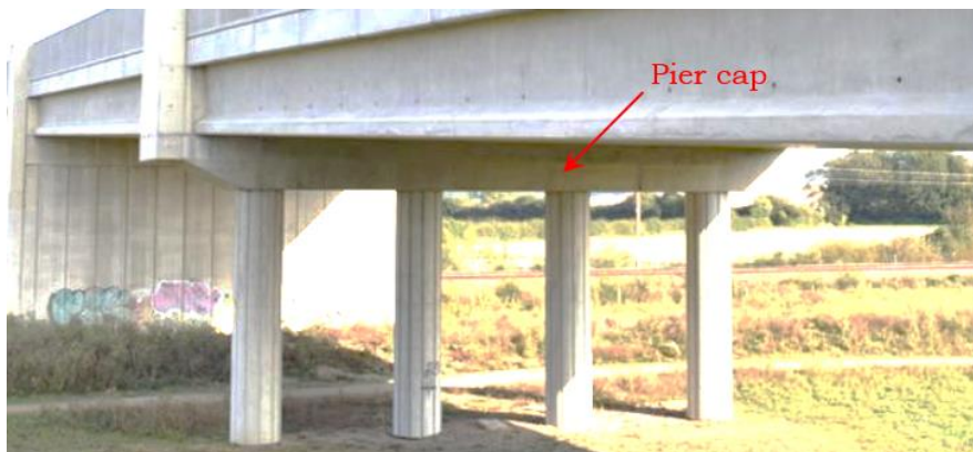
Figure 4.7 Location of a pier cap in a bridge
