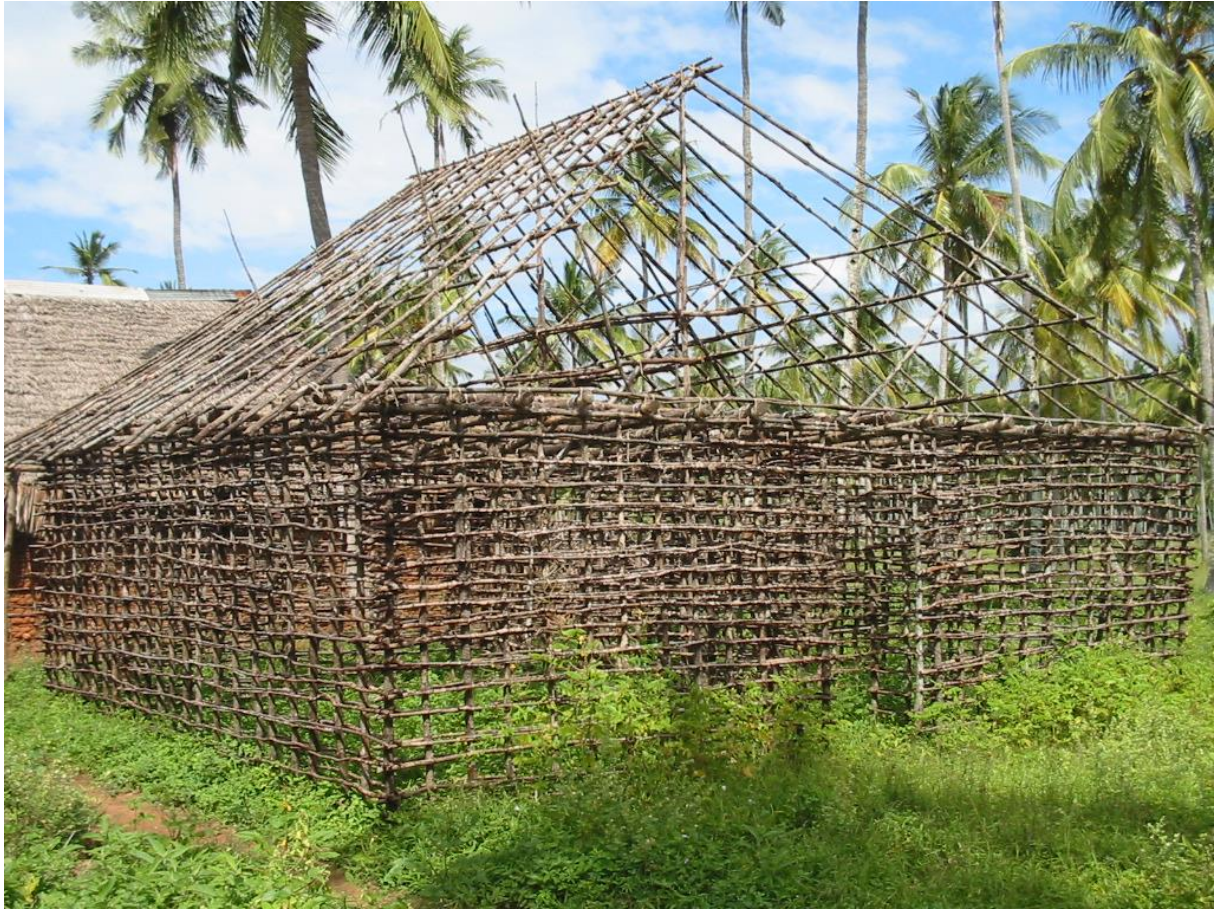
Figure S6. Typical Swahili house in Gazi Bay (Kenya) composed of poles from different mangrove species depending on their position in the construction. The Red mangrove Rhizophora mucronata is used for supporting pillars, the Yellow mangrove Ceriops tagal for the horizontal interweaving network and the Orange mangrove Bruguiera gymnorhiza for ceiling beams (Photograph by Griet Neukermans).
