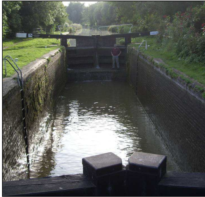
Figure 2. Interior of a typical lock. Note cill.
