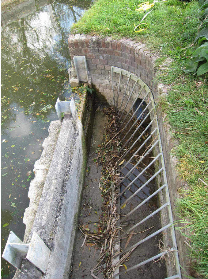
Figure 16. Example of complicated weir box.
