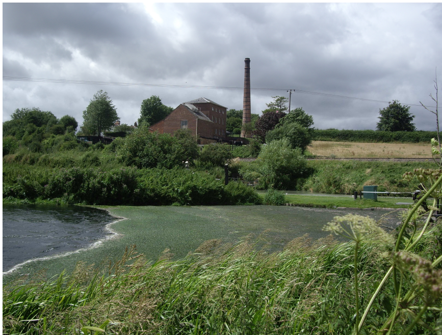
Figure 46. The outlet of Wilton Water Reservoir next to the Crofton Pumping Station. Note algal mat.
