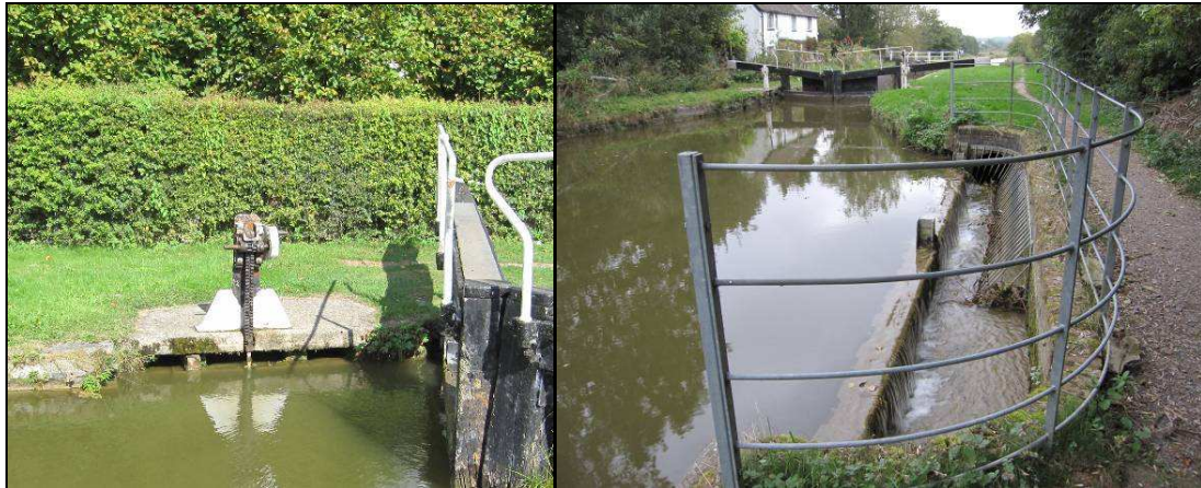
Figure 7. Typical overflow weirs on the Kennet and Avon Canal.
