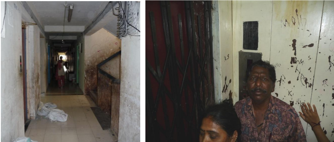
Figure 38 – Stairwells and lifts
