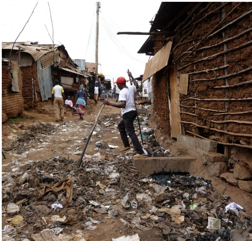
Figure 25 – Manual clearing of blocked open sewer
