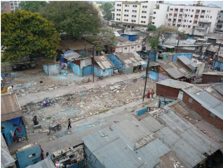
Figure 43 – Partly demolished adjacent slum
