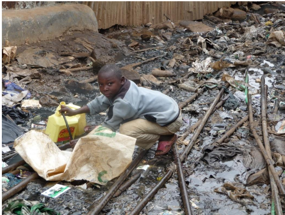
Figure 22 – Burst and contaminated water pipe lines
