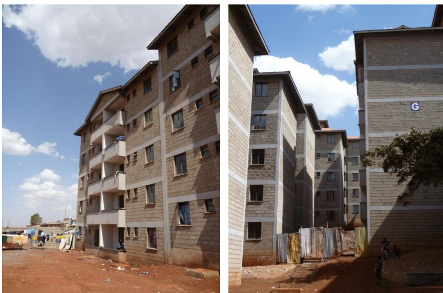
Figure 106 – Langata decanting site
