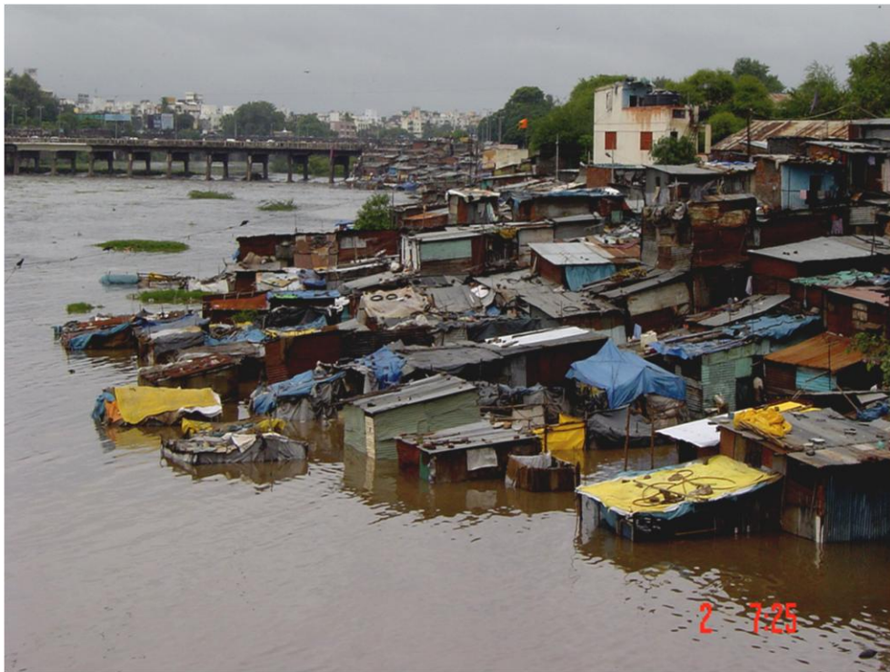
Figure 50 – The devastating floods at Kamgar Putala
