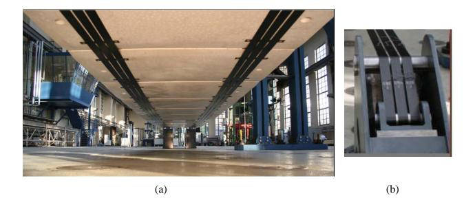
Figure 8. Stressed ribbon bridge (a) view from underneath the bridge (b) anchorage detail
