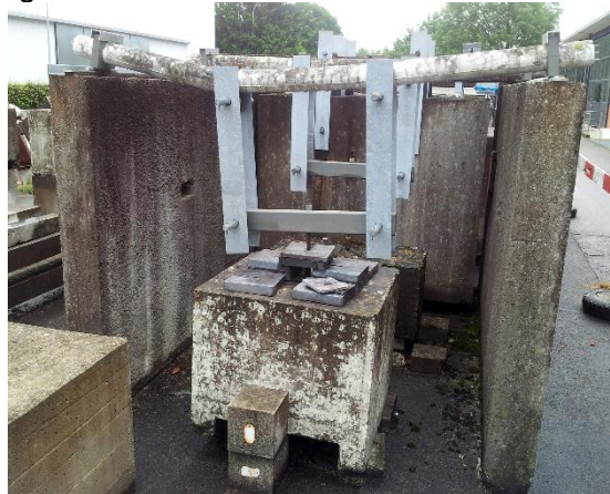
Fig. 10. Sustained loading test - failed CFRP prestressed spun concrete pole after 16.5 years of sustained bending
