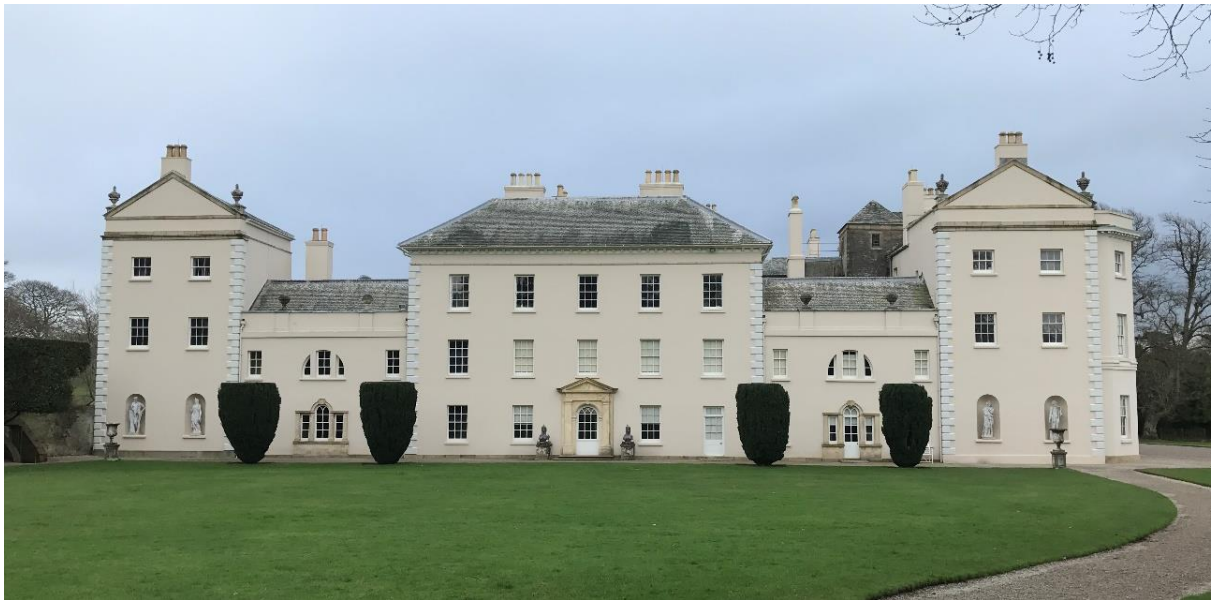
Fig. 3 Photograph of the west front of Saltram House.
