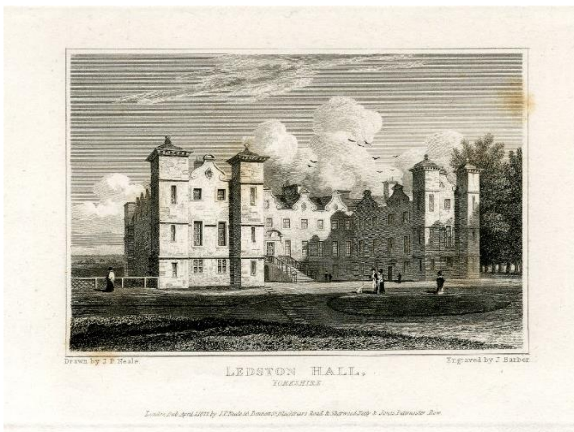
Fig. 6 Principal front of Ledston Hall, by John Preston Neale, 1822.
