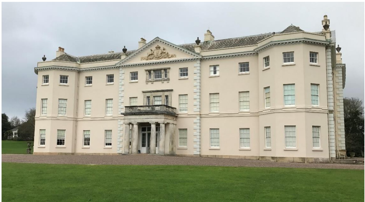
Fig. 2 Photograph of the south front of Saltram House.
