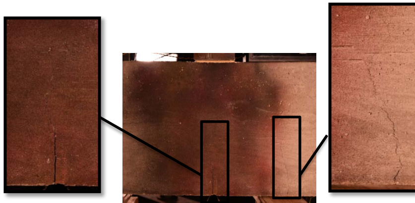
Figure 14: Cracks in beam M30,H220,0.4,FD
