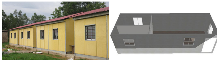
Fig 1. A typical commercially available low-cost modular house in India and its CAD model. [1]
