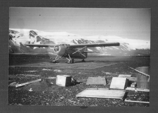
Plate 40. Test flying. Ski-wheel landing gear.
