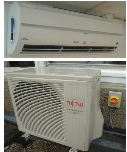
Figure 21.11. The inner and outer bits of an air-source heat pump that has a coefficient of performance of 4. The inner bit is accompanied by a ball-point pen, for scale. One of these Fujitsu units can deliver 3.6 kW of heating when using just 0.845 kW of electricity. It can also run in reverse, delivering 2.6 kW of cooling when using 0.655 kW of electricity.
