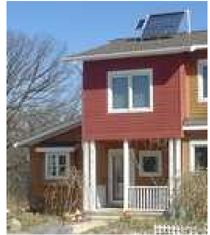
Figure 30.2. A solar water heater providing hot water for a family in Michigan. The system's pump is powered by the small photovoltaic panel on the left.
