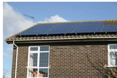
Figure 6.5. Solar photovoltaics: data from a 25\text{-m}^2 array in Cambridgeshire in 2006. The peak power delivered by this array is about 4 kW. The average, year-round, is 12 kWh per day. That's 20 W per square metre of panel.
