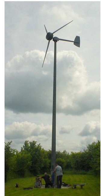
Figure B.10. A 5.5-m diameter Iskra 5 kW turbine [www.iskrawind.com] having its annual check-up. This turbine, located in Hertfordshire (not the windiest of locations in Britain), mounted at a height of 12 m, has an average output of 11 kWh per day. A wind farm of machines with this performance, one per 30 m × 30 m square, would have a power per unit area of 0.5 W/m 2 .
