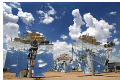
Figure 25.3. Stirling dish engine. These beautiful concentrators deliver a power per unit land area of 14 \text{ W/m}^2 . Photo courtesy of Stirling Energy Systems. www.stirlingenergy.com
