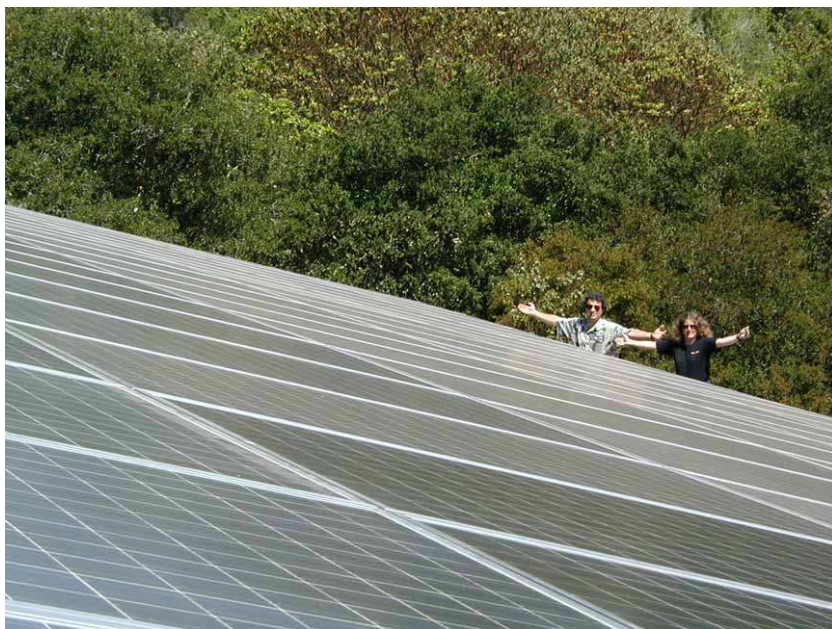
Figure 6.6. Two solar warriors enjoying their photovoltaic system, which powers their electric cars and home. The array of 120 panels ( 300\text{m}^2 each, 2.2\text{m}^2 each) has an area of 268\text{m}^2 , a peak output (allowing for losses in DC-to-AC conversion) of 30.5 kW, and an average output – in California, near Santa Cruz – of 5 kW ( 19\text{W}/\text{m}^2 ). Photo kindly provided by Kenneth Adelman.
