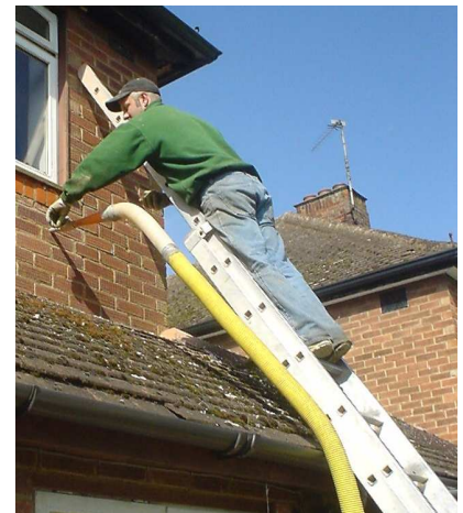
Figure 21.5. Cavity-wall insulation going in.
