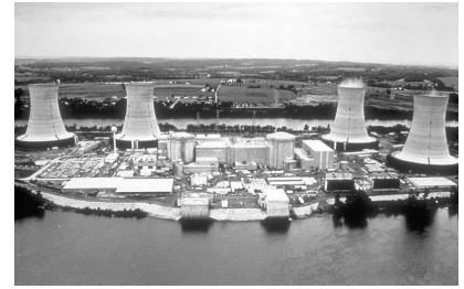
Figure 24.4. Three Mile Island nuclear power plant.
