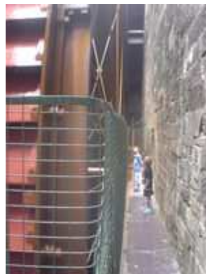
Figure 8.4. A 60 kW waterwheel.
