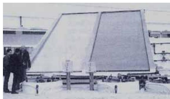
**Figure 1.11** Pilot scale TFFBR for textile wastewater treatment (Bahnmann, 2004)
