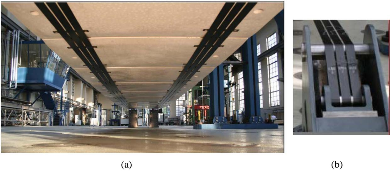
**Figure 8.** Stressed ribbon bridge (a) view from underneath the bridge (b) anchorage detail
