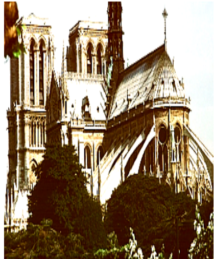
Fig. 8 Views of the apse and flying buttresses
