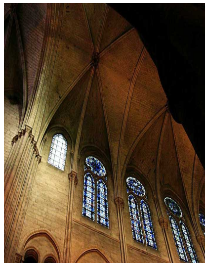
Fig. 12 Ribbed Vault
