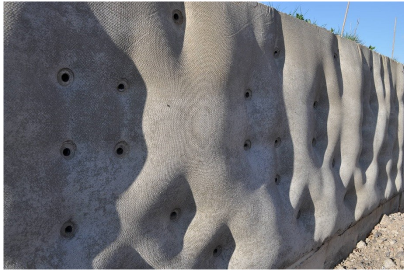
Figure 6 – Fabric formed retaining wall. Photo: Wilf Meynell/Studio Bark.
