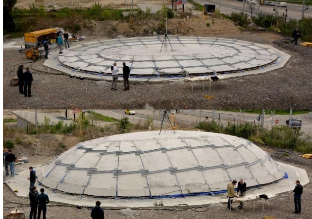
421 Figure 16 - Pneumatic forming of hardened concrete. Photo: TU Wien
