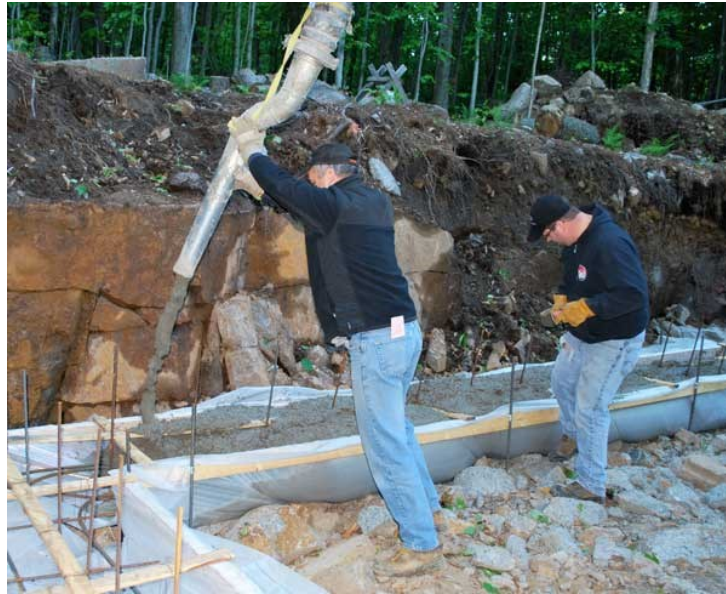
Figure 7 – Fabric formed strip footing. Photo: Fab-Form [25].
