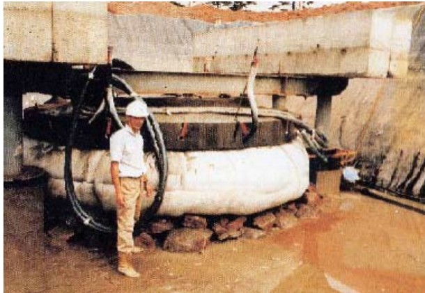
Figure 8 - Footing for precast marine structure. Photo: Proserve Ltd. [84].
