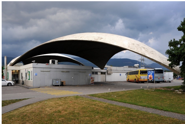
283 Figure 9 – Reinforced concrete canopy by Heinz Isler. Photo reproduced under CC-BY-SA/© Chriusha 284 (Хрюша) [88].
