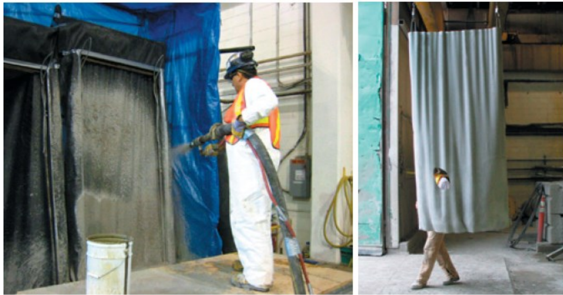
Figure 14 – Thin shell precast wall panel created with sprayed concrete. Photo: Mark West (C.A.S.T.) [49].
