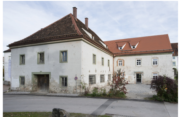
Figure 1 The Alte Schäfflerei building at the Fraunhofer Centre. Different internal wall insulation systems using CDD as a separating layer are being tested in the upper floor. Photo: Fraunhofer IBP.
