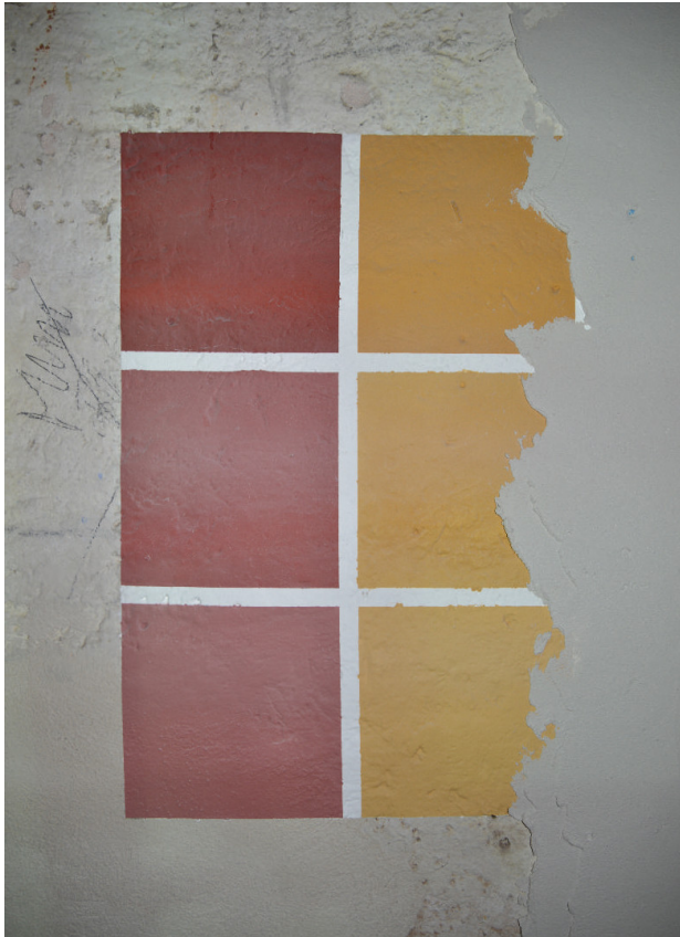
Figure 3 A test matrix with different colour binding systems. The test squares have been sprayed with CDD and are already partially covered with the reversible plaster layer. Photo: Fraunhofer IBP.
