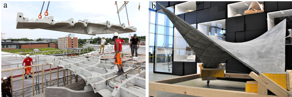
Figure 2.5: Examples of innovative forming methods for concrete, including a) a ribbed post-tensioned floor slab using 3D printed formwork (image by Tom Mundy, copyright Digital Building Technologies, with permission) and b) hybrid flexible formwork using a cable-net and fabric described by Veenendaal and Block (2014) (image courtesy Diederik Veenendaal, BRG, ETH Zürich).
