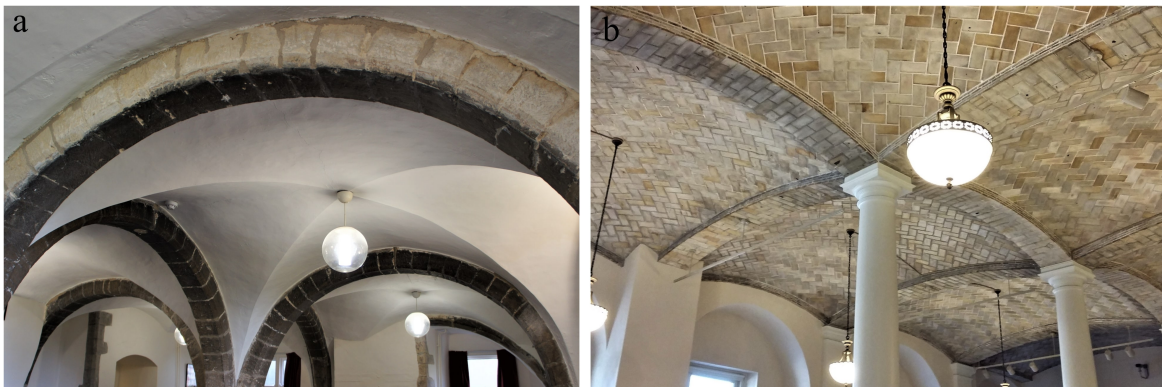
Figure 1.3: Historical example of vaulted floors using brittle materials, including a) masonry undercrofts constructed in the 12th century for the monastery of Ely cathedral and b) tile vaulting in the Boston public library, constructed by Raphael Guastavino in 1895.
