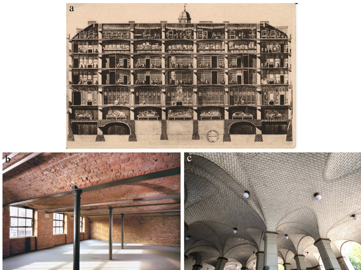
Figure 2.2: Examples of tile and brick vaults in fireproof multi-storey buildings, including a) the Office of Foreign Affairs and the Navy in Versailles (photo gbaudouin4, licence: CC BY-NC-SA 2.0), b) Waulk Mill in Manchester (image copyright Urban Splash with permission) and c) the entrance to the City Hall subway station in New York (photo Emil Adiels, licence: CC BY-NC-ND 2.0).
