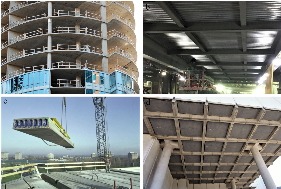
Figure 1.1: Typical multi-storey floor structures including a) reinforced concrete flat slabs (photo by Darren Kirby/CC BY-SA 2.0), b) steel composite decking (photo by MTA Capital Construction Mega Projects/CC BY 2.0), c) pre-cast hollow core concrete units (photo by Michael Schmah/CC BY-SA 2.0) and d) waffle slabs (photo by Peka/CC BY-SA 4.0).
