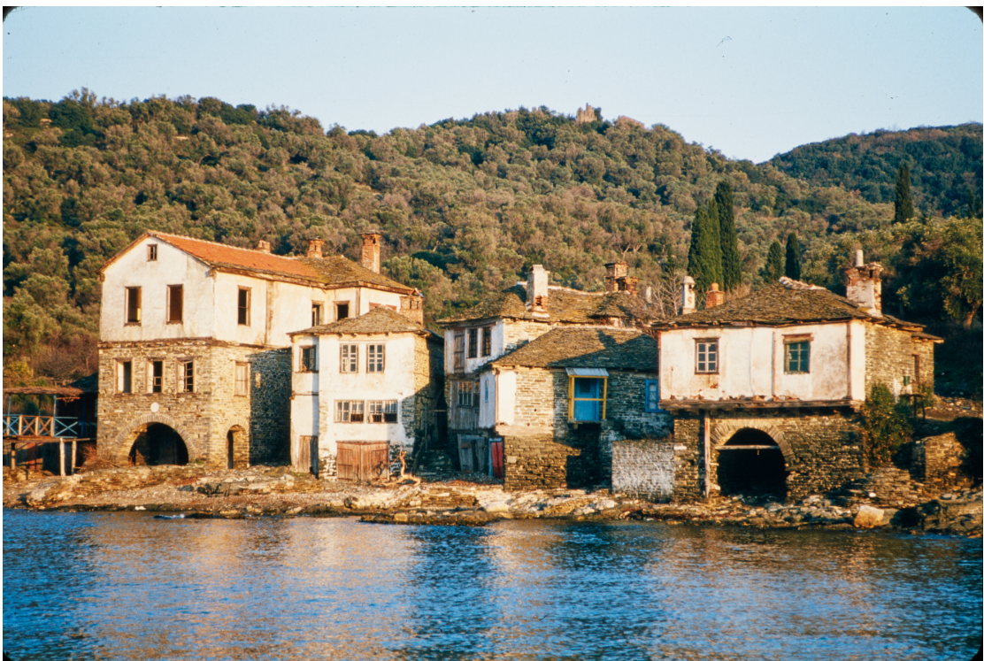
[17] Vatopedi Monastery, boathouses and accommodation for lay workers. (February 1987)
