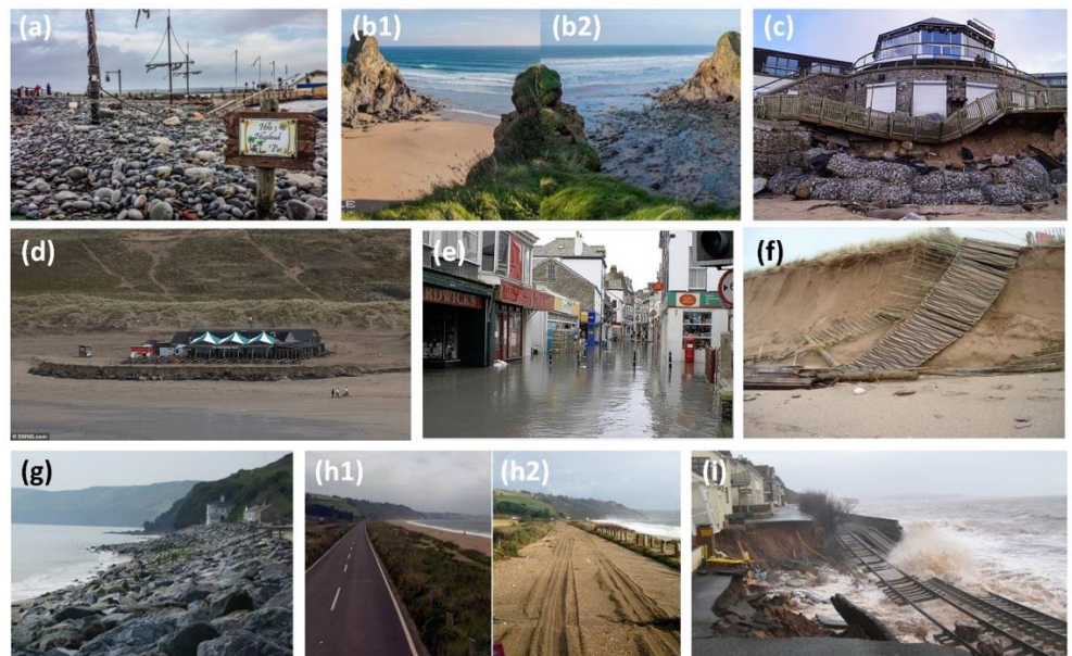
Figure 2: Pictorial overview of storm impacts along the coast of south-west England (from Scott et al. , 2016). (a) The gravel barrier at Westward Ho!, north Devon, experienced overwash during the spring tide of 2/3 January 2014, resulting in the deposition of a large amount of pebbles and cobbles into the local mini-golf course located just behind the ridge. (b1 before; b2 after) The significant storm ‘Hercules’ on the 5th January 2014 removed large quantities of sand from at Whipsiderry beach, north Cornwall, exposing the underlying rocky shore platform. (c) Hercules caused extensive damage to coastal infrastructure along the north Cornish coast; here the seawall below Fistral Blu bar in Newquay collapsed and damaged the property. (d) The Watering Hole in Perranporth, North Cornwall, the only ‘beach restaurant’ in the UK, required human intervention to ensure the restaurant remained high and dry after winter storms lowered the beach by several meters. (e) The coastal town of Looe, south Cornwall, got flooded a number of times during the 2013/2014 winter. (f) The coastal dunes at Thurlestone, south Devon, experienced more than 5 m of erosion during the 2013/2014 winter resulting in the collapse of the wooden boardwalk. (g) At the end of the winter, the beach in front of the seawall at Beesands, south Devon, had completely disappeared. (h1 before; h2 after) The road that runs
