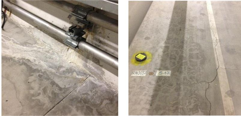
**Figure 3.20.** Water leakage with calcite deposits (close to magnet QID 101100).
