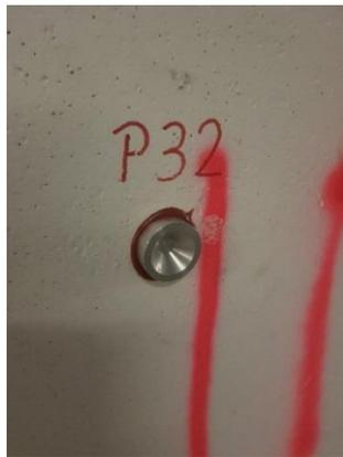
**Figure 3.26.** Geodetic bolt installed on tunnel lining.
