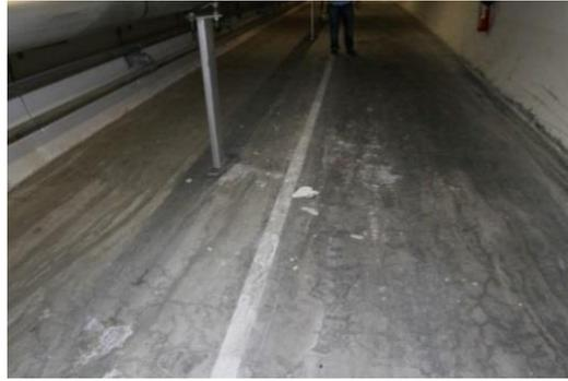
**Figure 3.13.** Concrete flaking from tunnel crown.
