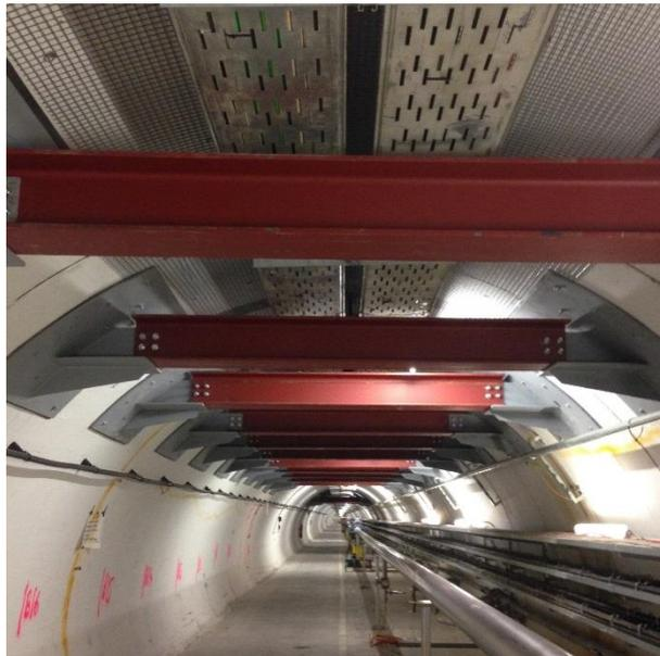
**Figure 3.24.** Installation of steel I beams in the critical area along the TT10 tunnel between magnets QID 101300 and QID 101400.
