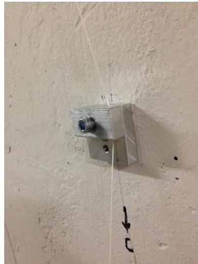
**Figure 4.17.** Metallic clamps for attaching the FO cable to the tunnel lining.
