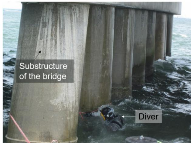
**Figure 2.7** A diver carrying out an underwater bridge inspection (Diving Services Inc., 2017)
