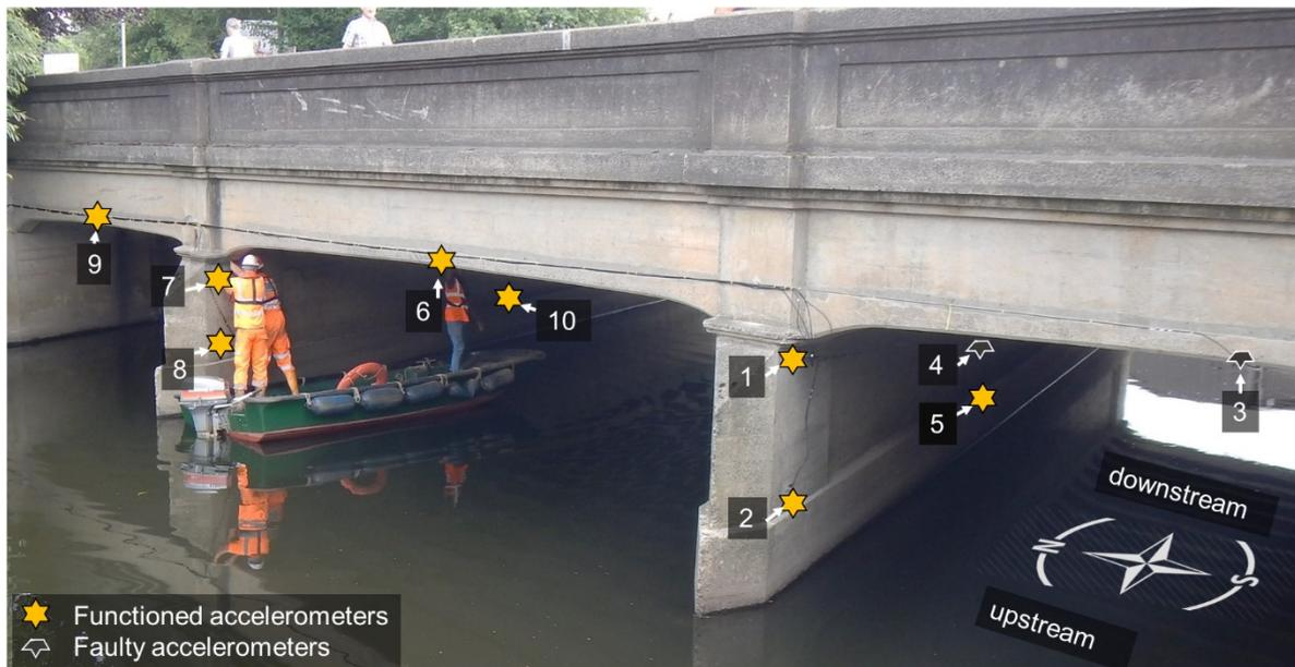
**Figure 3.12** Arrangement of accelerometers at Baildon Bridge
