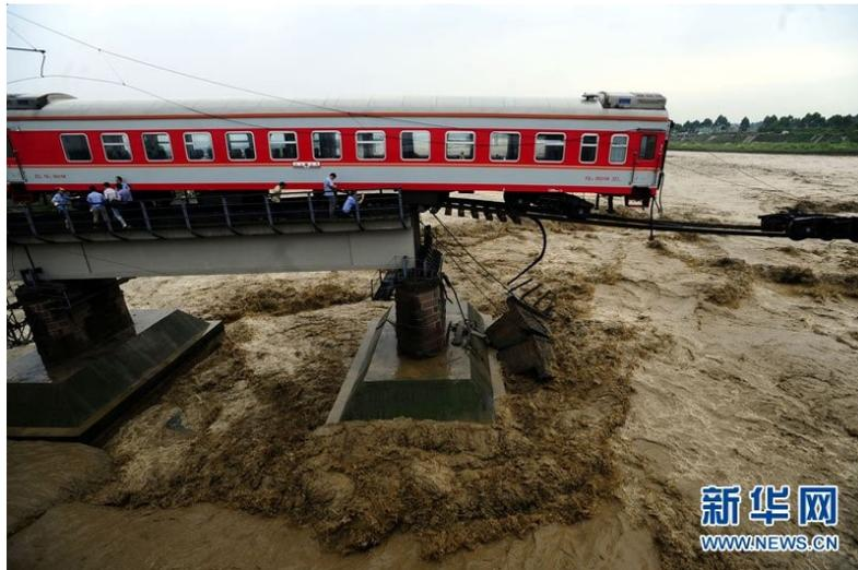
**Figure 2.4** *Shi-Ting-Jiang Bridge failed because of scour in 2010 (CNTV, 2010)*
