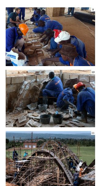
Figure 9. Rwanda Cricket Stadium training: joining two tiles Figure 10. Rwanda Cricket Stadium training: building small vaults Figure 11. Rwanda Cricket Stadium building the edge arches
