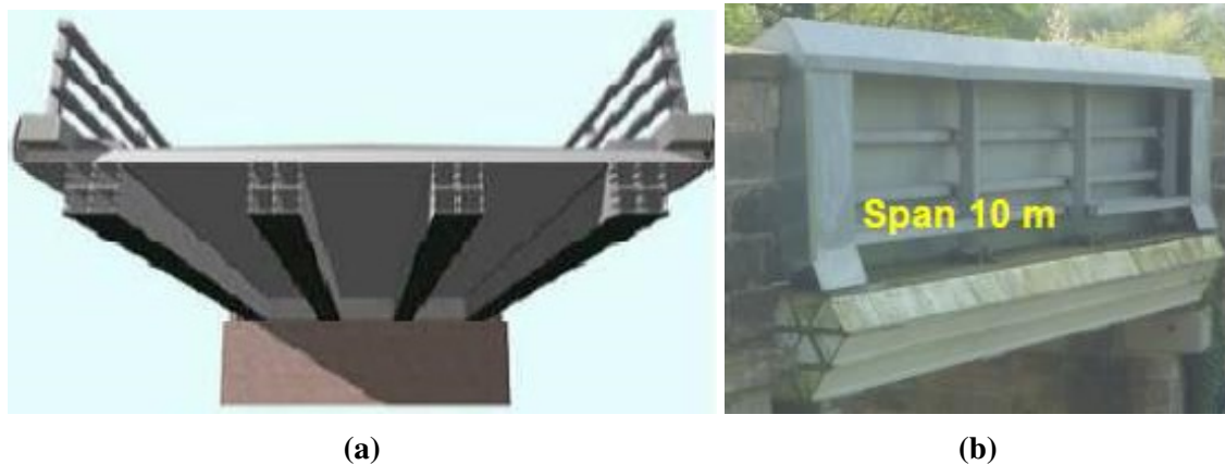
Fig. 1.15 (a) Typical cross section of the West Mill Bridge [17]. (b) Standen Hey road bridge uses GFRP deck pultrusions laid span-wise [18].
