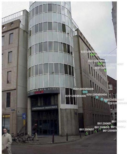
Figure 8.20 Façade with monitoring points Rokin 65 seen from Rokin Station side (Rokin)
