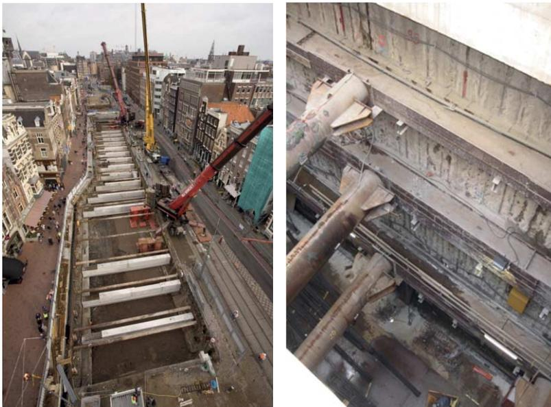
Figure 4.16 First excavation (left) and strut layers (right)
