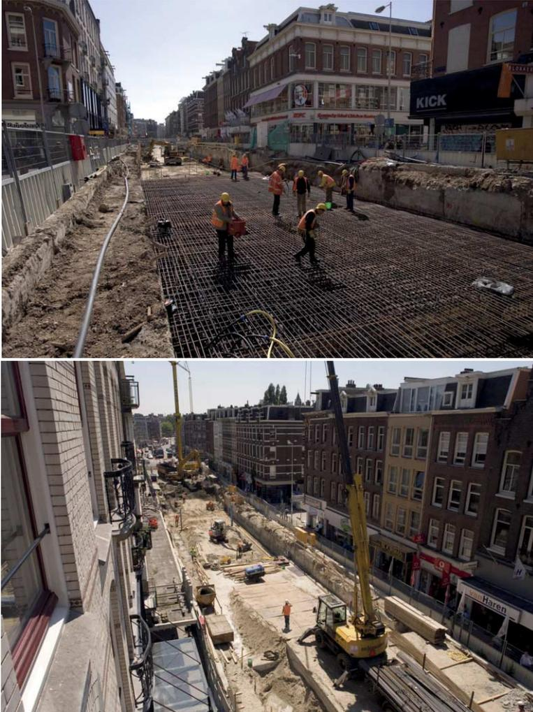
Figure 4.29 Construction of the roof (top) and back fill above the roof (bottom)
