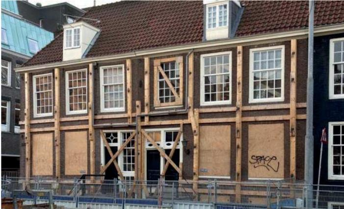
Figure 10.6 Damaged buildings Vijzelgracht 20-26 due to first incident June 2008
