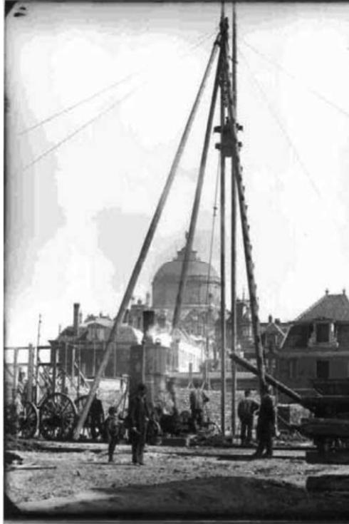
Figure 4.5 Installation of wooden pile by steam engine (picture taken in 1891 by Jacob Olie)
