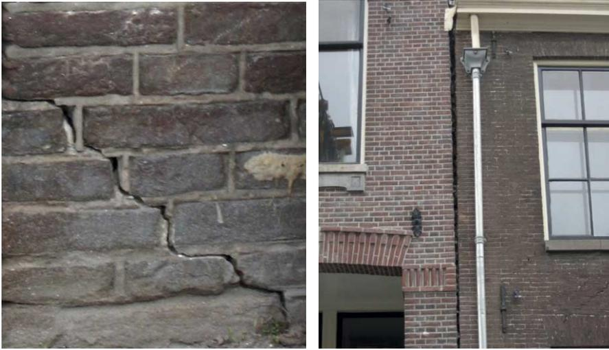
Figure 2.16 Crack due to shear deformation (left) and relative rotation of one building to the other (right)
