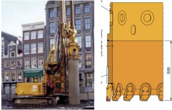
Figure 4.14 Equipment for removal of obstacles with large diameter drilling
