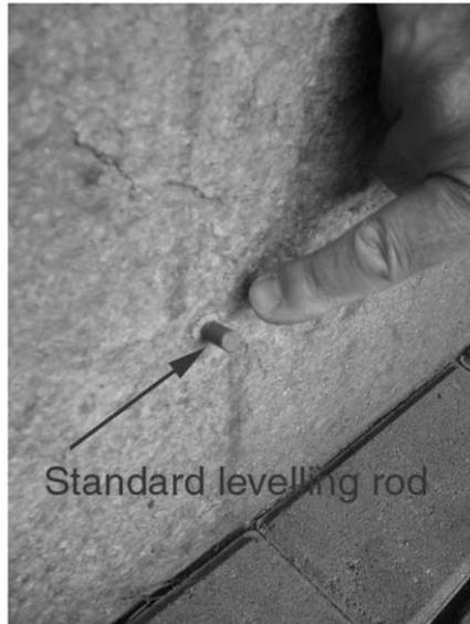
Figure 4.33 Manual levelling point
