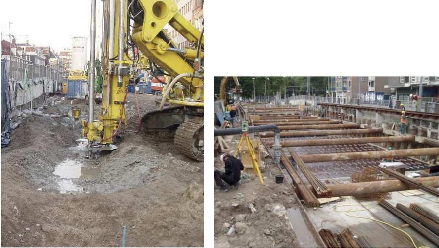
Figure 4.22 Installation of the jet grout strut (left) and construction of the roof (right)
