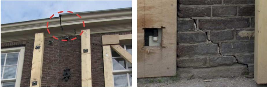
Figure 10.9 Details of cracks; left: crack 1, width max. 20 mm, right: crack 4, width max. 8 mm.
