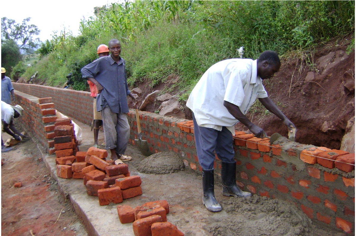
Figure 15: Suam villagers employed to construct the channel for MHP Suam
