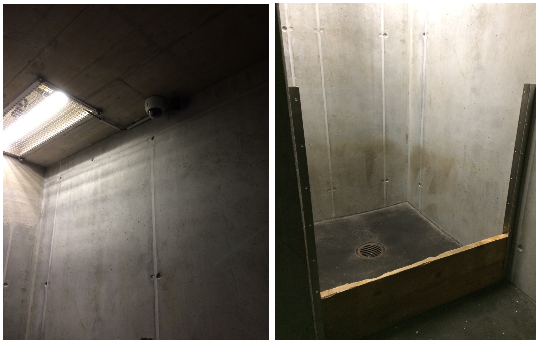
Fig.51 The maternity den constructed in the Tiergarten Schönbrunn in Vienna, complete with CCTV, drainage (for cleaning out of season), and microphones to pick up cub/mother vocalizations, (H. Anderson-Elliott, 2018)
