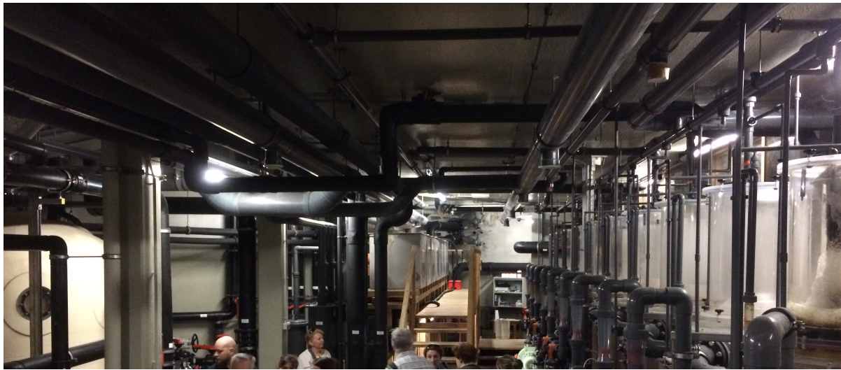
Fig.59 The primary underground water filtration and pump room of the Vienna Schönbrunn polar bear enclosure, (H. Anderson-Elliott, 2018)
