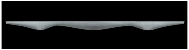
Figure 8 Fabric-cast concrete 'bending moment' beam (courtesy of Mark West)
