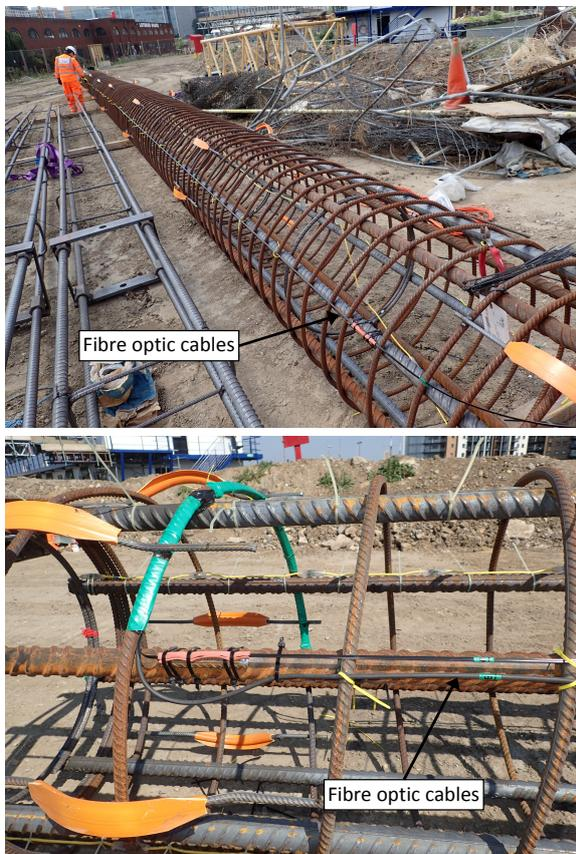
**Figure 2.** Distributed fibre optic sensor cables being installed on the reinforcement cage of a CFA pile (top) and wrapped around the bottom of the cage (bottom).
