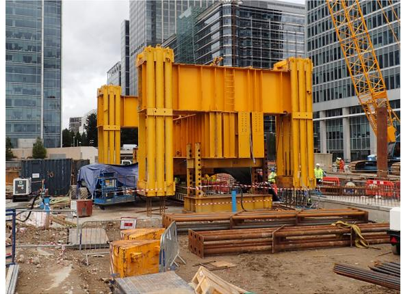
**Figure 1.** Static load testing frame for a trial test pile.
