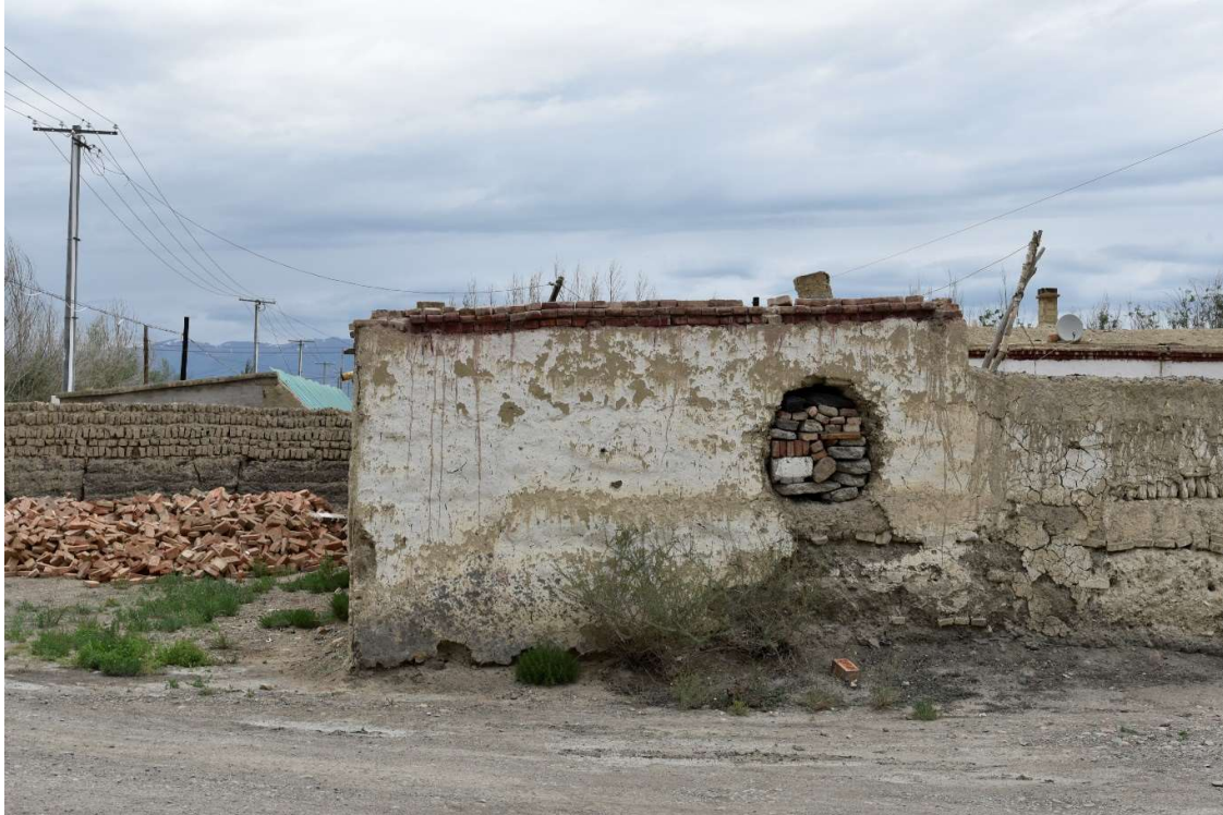
Figure 4: A so-called ‘tufang’ dwelling with wall partially revealing it as a brick structure and earthen covering.
