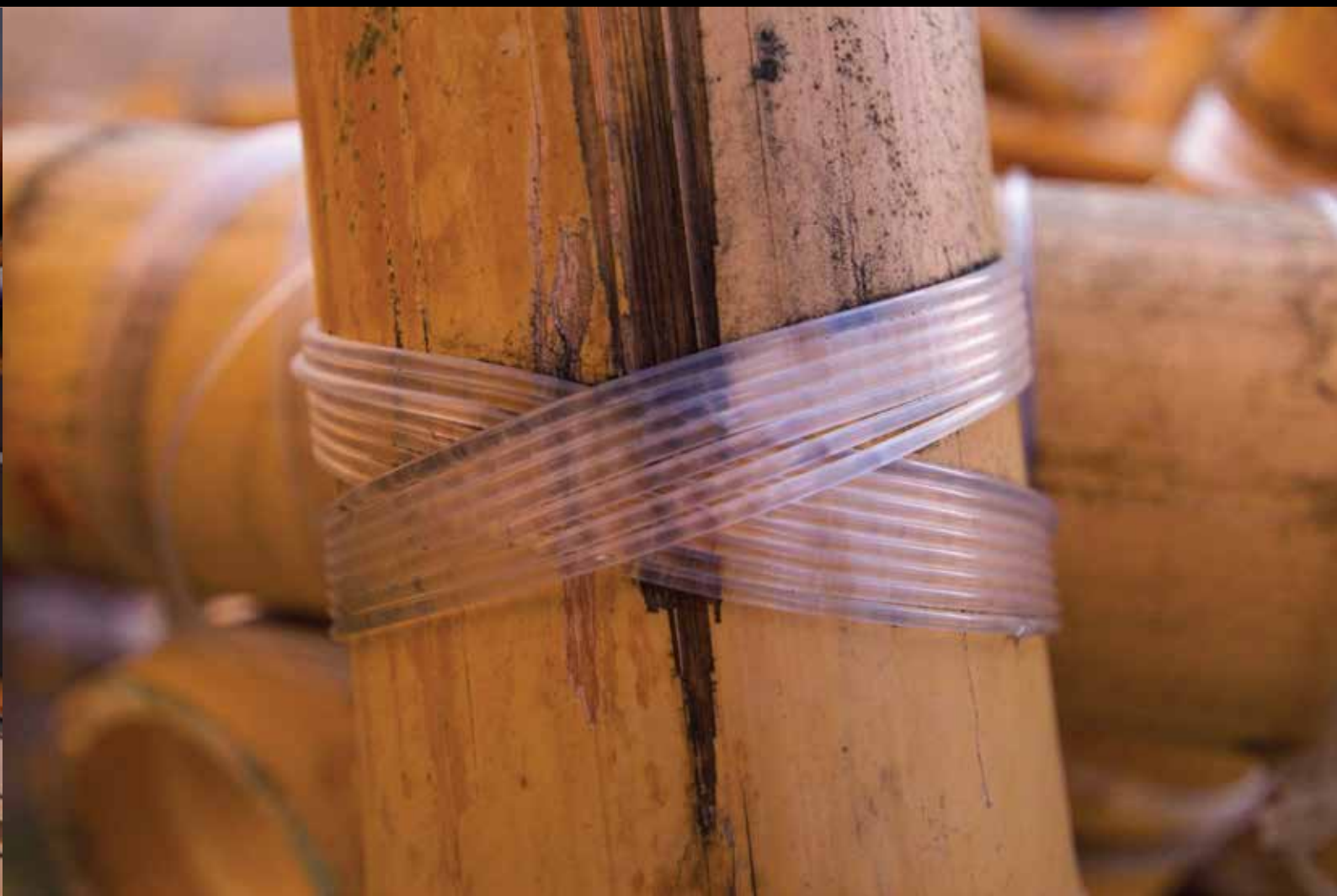
Image 24: Diagonal lashing. July 2014. Department of Architecture. Cambridge
