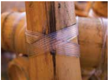
Image 15: Diagonal lashing
