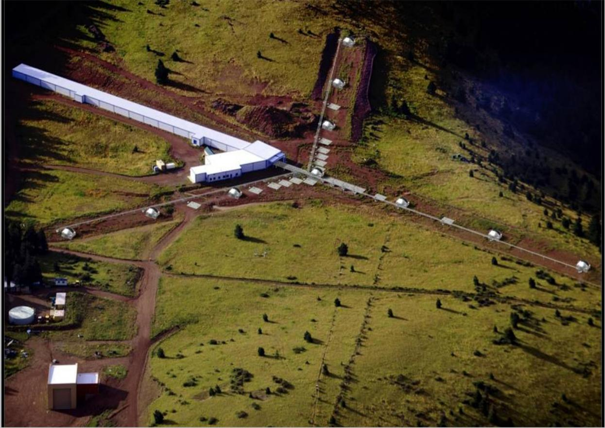
Figure 1: Photo of the completed MROI beam combining facility taken Fall 2015. In the lower left of the foreground is the Visitor's Center and Maintenance Facility where telescope mount #1 is currently undergoing Site Acceptance Testing. Overlaid on the photo of the array are superimposed pads, telescopes and a beam relay system rendered by lead opto-mechanical MROI engineer A. Olivares and based on the actual design of the MROI infrastructure. The photo of the site courtesy of T. Eakman.
